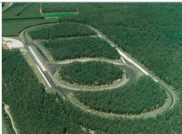
75,000 square meters of land was cleared for the new test track
